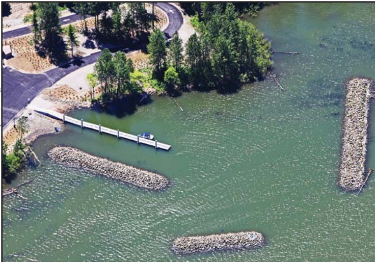
Rock Breakwaters / Wyeth, Oregon
