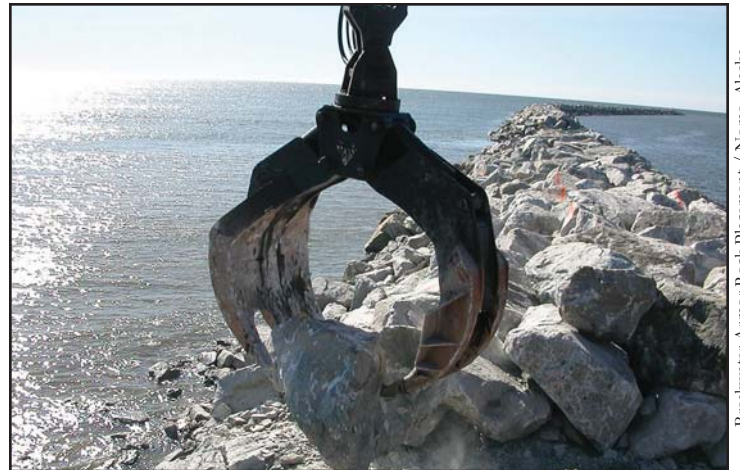
Breakwater Armor Rock Placement / Nome, Alaska
